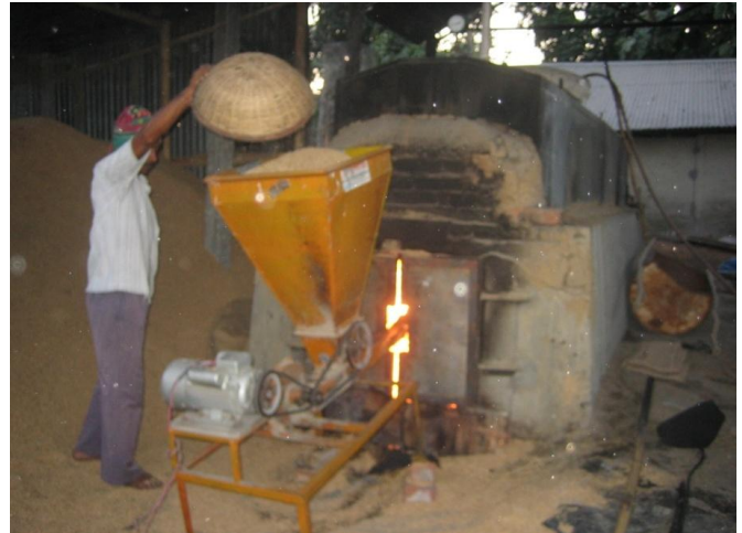
Fig. 4. Improved rice parboiling boiler
